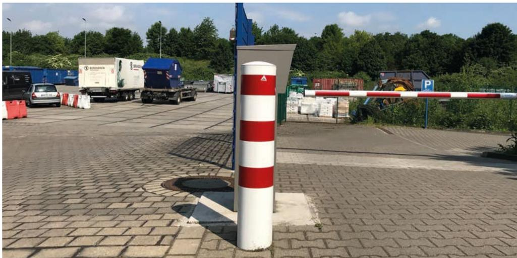
**BORNE EN TUBE D'ACIER Ø 273 X 5,0 MM**
